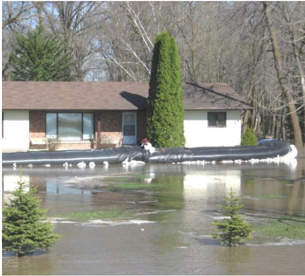
Figure 9. Water filled dams protecting a house from flood water The water filled dams also prevented property and other structures from flood water damage. Figure 9 shows water filled dams around the perimeter of a house defending flood waters.
