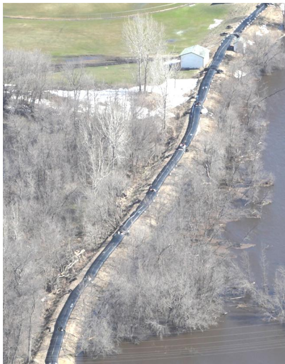
Figure 7. Water filled dams providing extra freeboard over an existing earthen berm.
