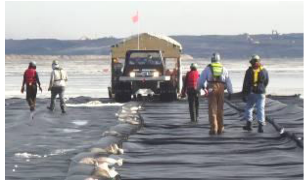
Figure 4. Placement of geotextile on frozen tailings pond.
