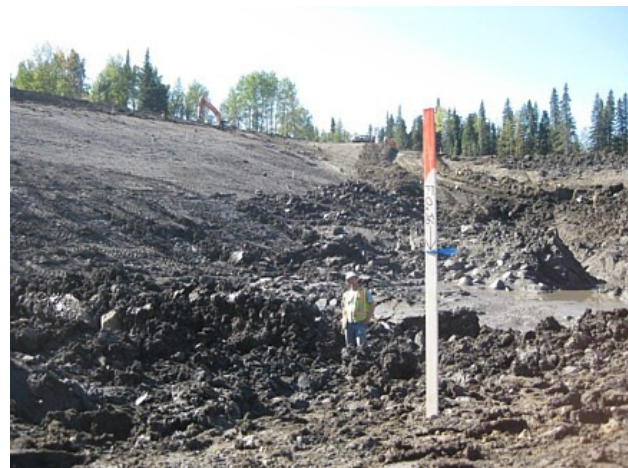
Figure 5. Subgrade preparation in wet conditions.
