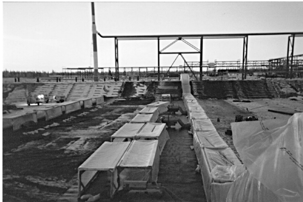
Figure 3. HDPE installation using temporary shelters.
