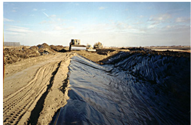
Figure 2. RPE irrigation canals in the winter in Alberta
