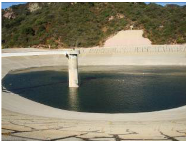
Figure 4 and 5: Original reservoir (left) and after removal of tower and new asphalt lining (right). Note the original concrete lined slope at back.
