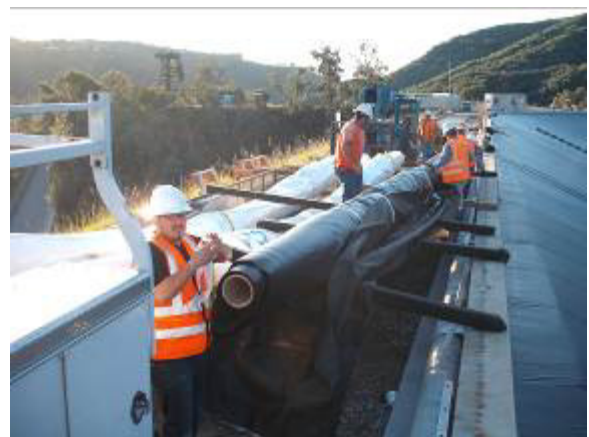
Figure 8: Installing a 35 ft wide fabricated panel.
