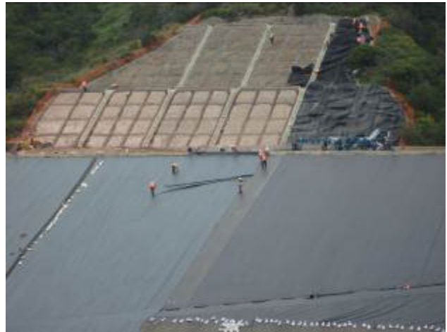
Figure 9 and 10: Chafer strip installation (left). Cover panels being installed (right).
