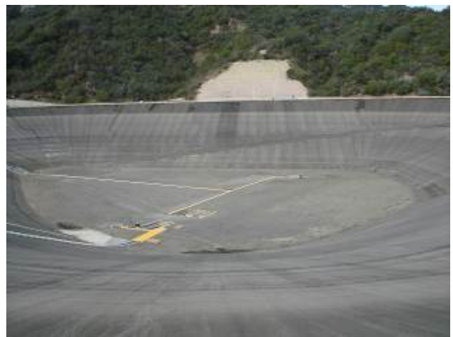
Figure 4 and 5: Original reservoir (left) and after removal of tower and new asphalt lining (right). Note the original concrete lined slope at back.
