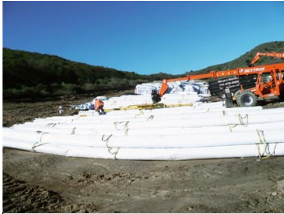
Figure 4: 36 ft wide prefabricated liner panels
