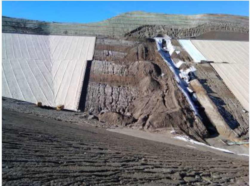
Figure 6: Subgrade damage after a significant rainfall event.
