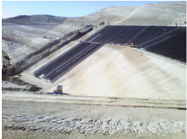
Figure 3: Placement of the geocomposite underdrain.
