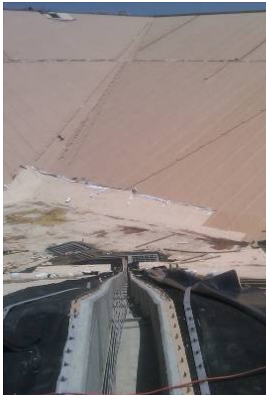
Figure 7: Pneumatic tubing in concrete trough
