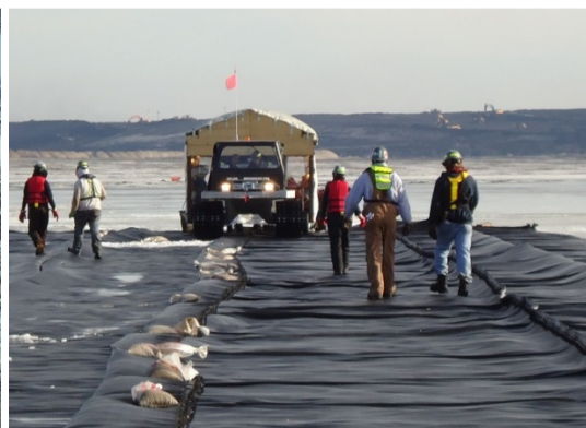
Figure 7. Fabric placement on ice.
