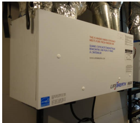
8. A heat recovery ventilator (HRV).
