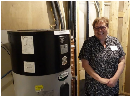
2. An air source heat pump water heater.
