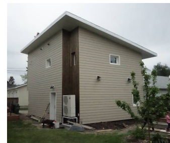
3. An air source heat pump unit on a garage suite.
