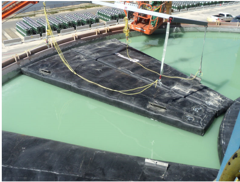
Figure 4 200 mm thick insulated cover on an acid clarifier.
