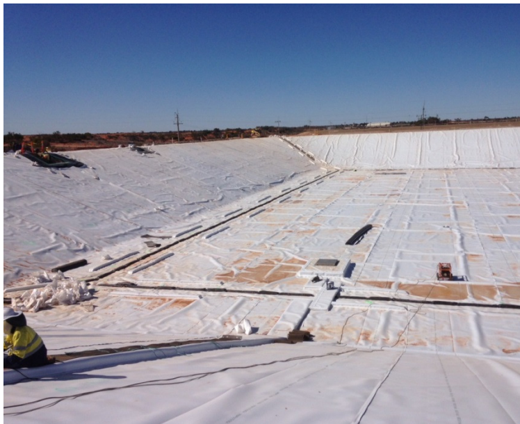
Figure 2 Fortified floating cover material at a mine site in Australia
