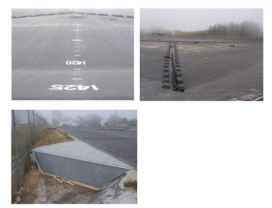
The final step in the construction of a potable water reservoir is to inflate the cover with air for cleaning and disinfection. We build special hatches on the cover that can accommodate blower fans for inflation. Once the fans are placed the cover is inflated so that workers can get underneath. A final cleanup of the space between the liner and the
