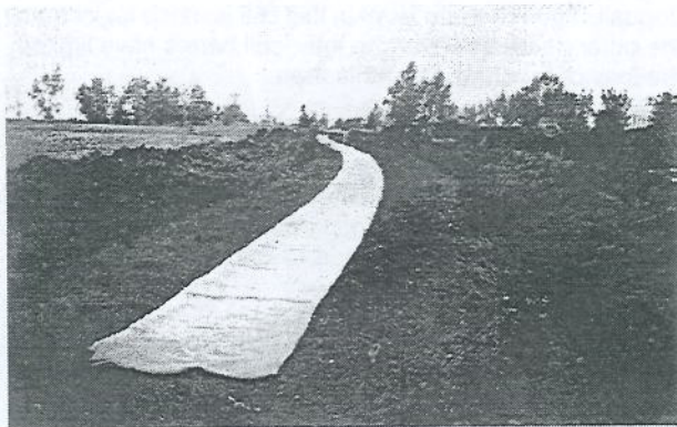
Figure 5 Deployment of the PVC geomembrane in the channel. View is looking north along swale.
