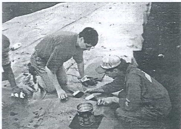
Figure 6 Welding panels of PVC together with solvent.
