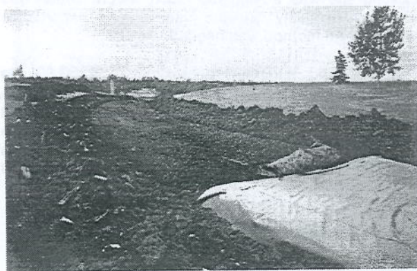
Figure 4 Channel looking toward the river. Excavated waste is visible along the left side of the channel.
