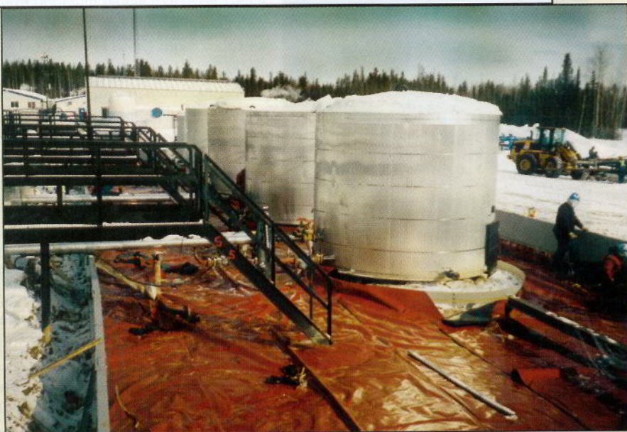
Photo 1: This secondary containment system uses a portable steel dike system with a polyurethane geomembrane.
