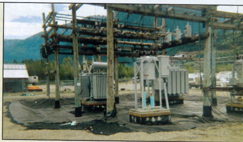
Photo 3: Oil-filled transformers, like those found at this electrical substation, often utilize small secondary containment geomembranes.
