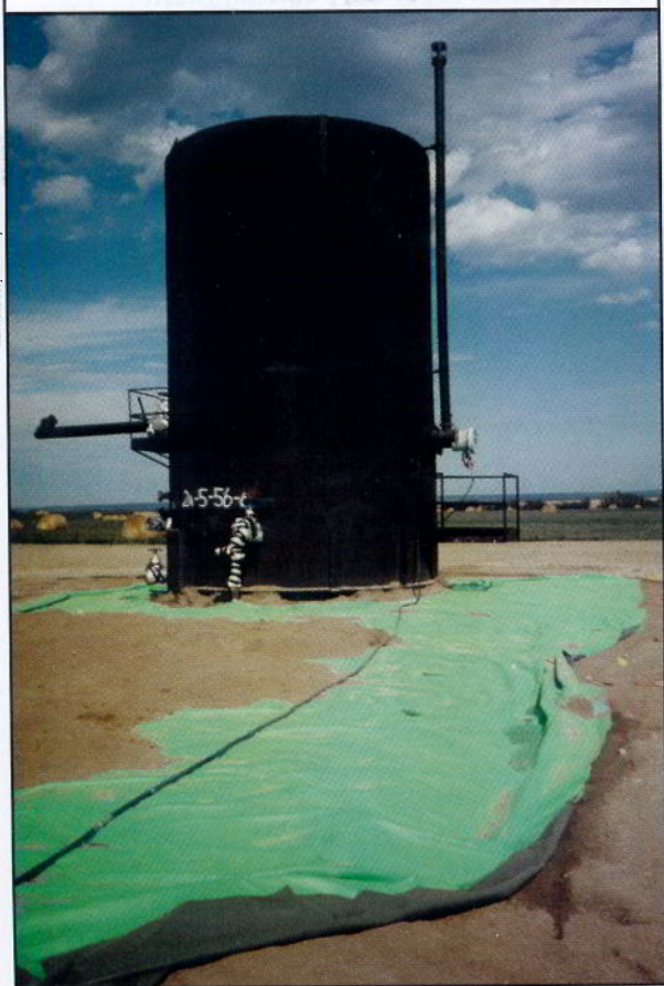
Photo 4: The tank at this oil well is being fitted with a PVC alloy geomembrane engineered for hydrocarbon resistance. In this case the liner was placed, and the tank set before the dike walls were built.
